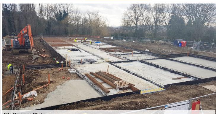
Site Progress Photo Site photo showing the progress to the foundations, pop-up drainage, and floor slabs.
